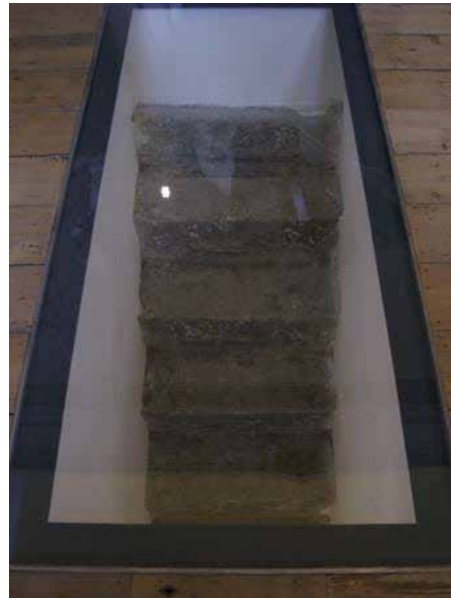
Recently uncovered flight of granite steps leading to holding cells in the basement.
