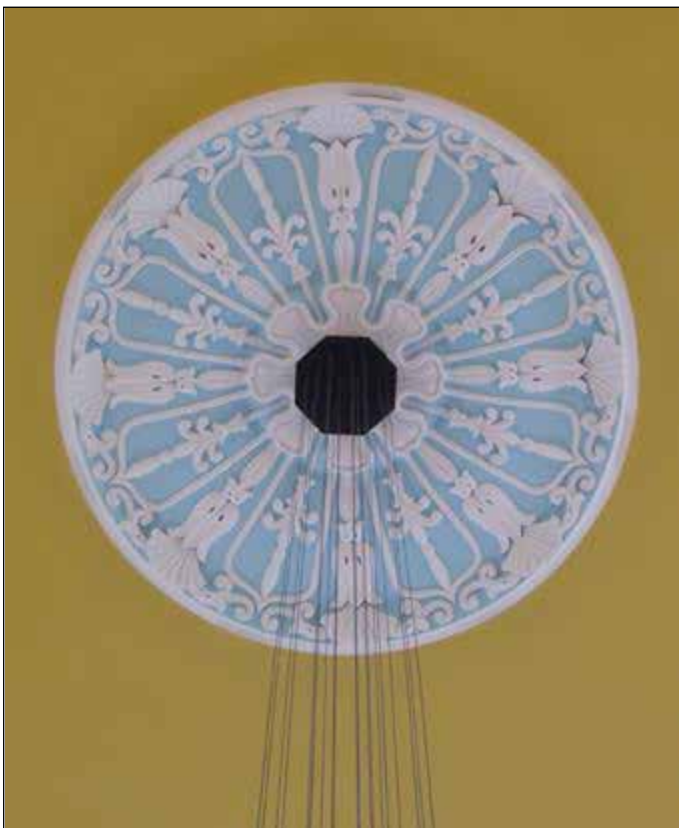
Restored Ceiling Rose and new light fitting .
