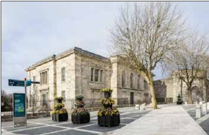
Kilmainham Gaol Courthouse
